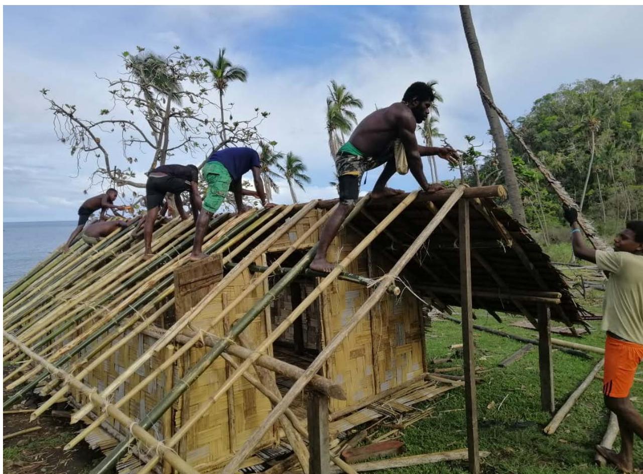
Vanuatu Tropical Cyclone Harold - Rebuilding houses Credit: VBRC / Glen Craig
